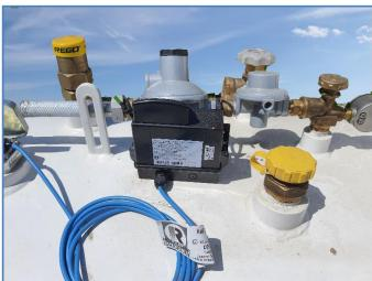
The device is ATEX approved and via the installed SIM Card the device is sending the data to a platform called "Tank Monitoring" used by the LPG companies and the corresponding haulers.
