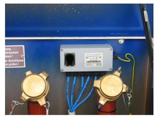
Practical example Installation of a SECU Multiplexer in the filling shaft
